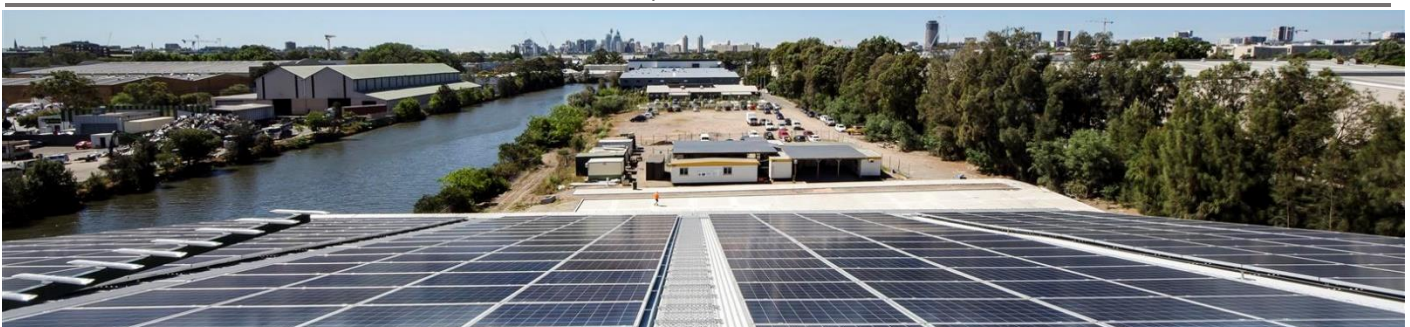
Alexandria Canal Depot: PV Solar Installation
